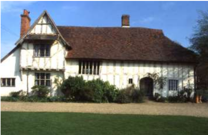
An English medieval farmhouse, made from small oak-trees, carpenter's oddments, reused oak timbers, elm and ash, and coppice poles.
